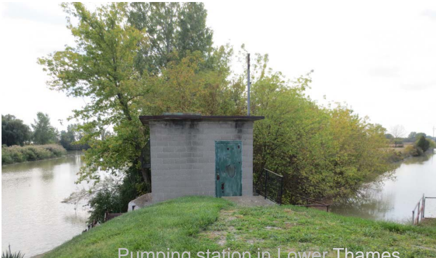
Pumping station in Lower Thames
