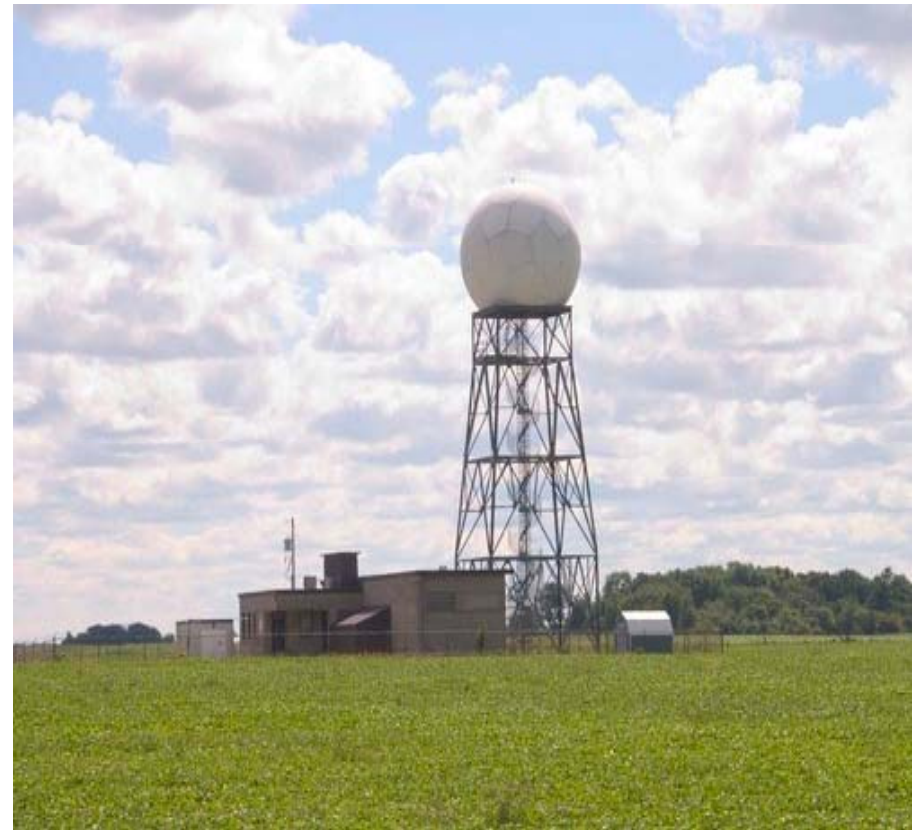
Exeter Radar Station (Environment Canada)
