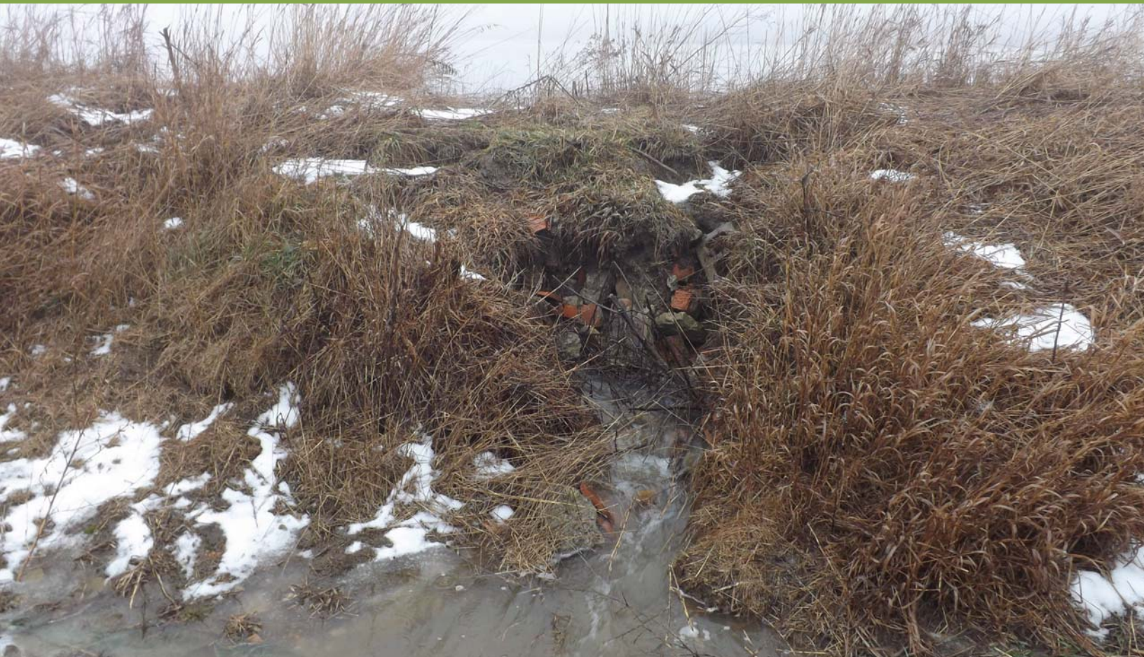
Existing Terrace Breach
